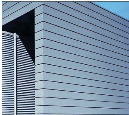
④ HORIZONTAL LAP SIDING
