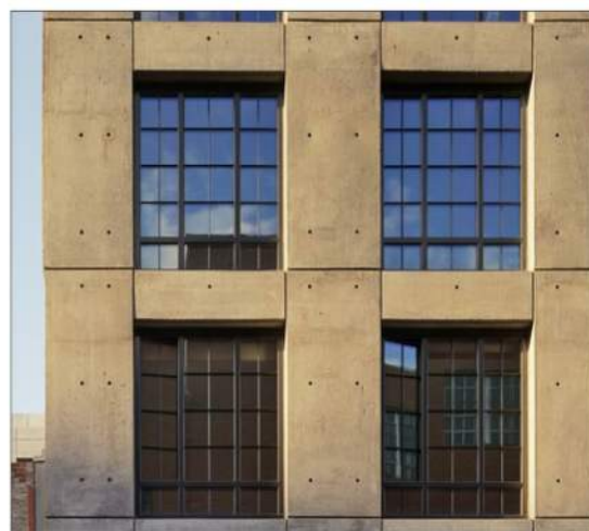
12 PRECAST CONCRETE PANELS
