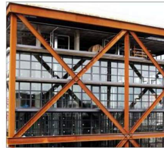
9 STRUCTURAL STEEL FRAME
