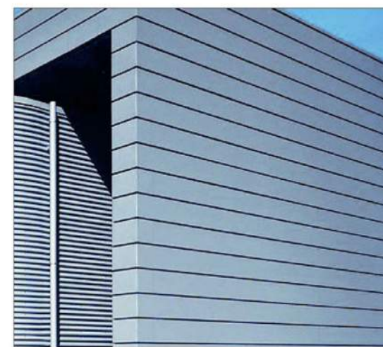
4 HORIZONTAL LAP SIDING
